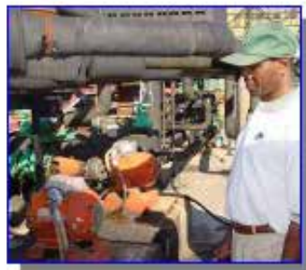
Upgrades to hotel chiller units
