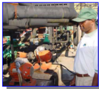
Upgrades to hotel chiller units
