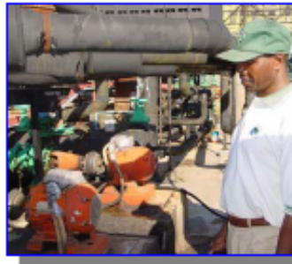
Upgrades to hotel chiller units
